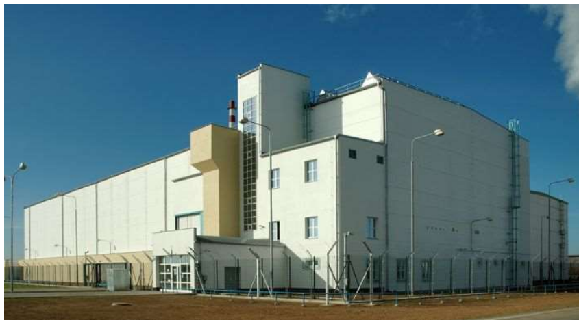
Fig. D 3 Interim Spent Fuel Storage Dukovany NPP
