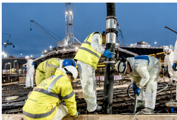
Concrete pouring at Hinkley Point C © EDF Energy
