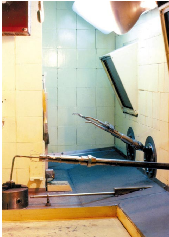
Figure 1.8 The manipulators that are used in the semi-hot chamber for handling the sources
