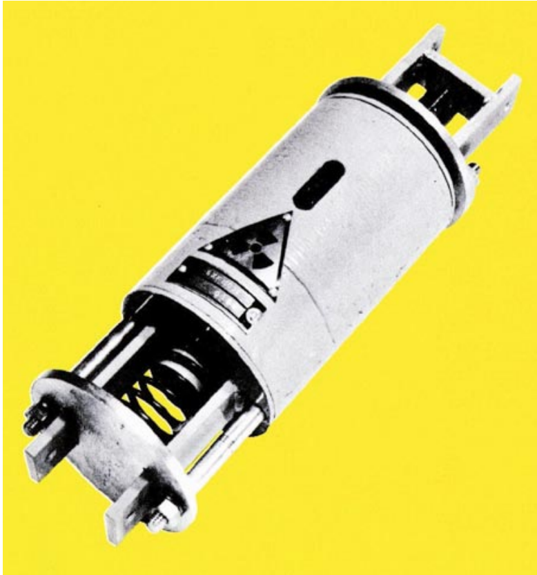
Figure 3.5 MDG-201 – the shield is intended to be assembled into protective tubes. Used with ^{60}\text{Co} , activity up to 700 MBq (but with additional thick shield). Produced by Tesla Liberec. From the company documentation of the former Tesla Liberec
