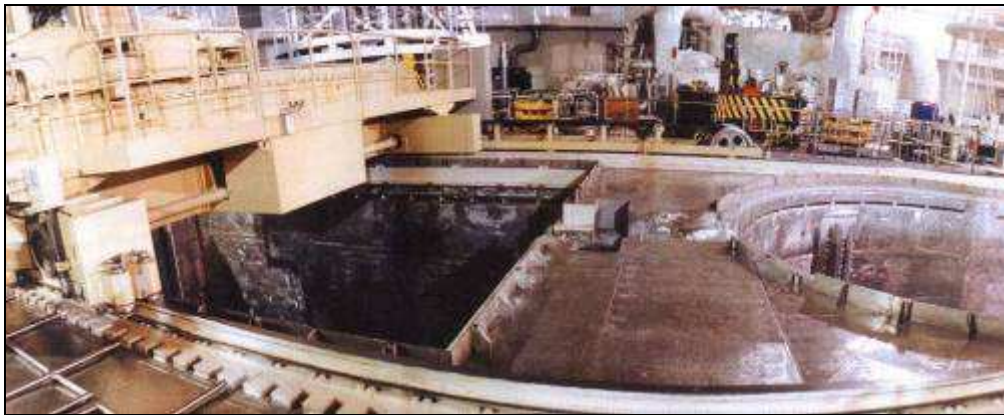
Fig. 4.3 Uncovered SF pool at NPP Temelín
