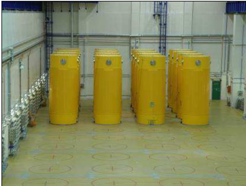
Fig. 4.4 Storage hall in SFSF Temelín
