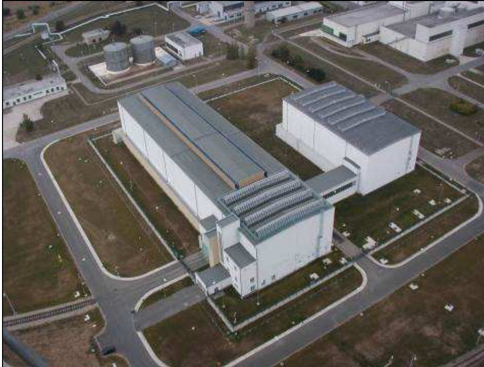
Fig. 7.1 View of SFSF Dukovany (left) and ISFSF Dukovany (right)
