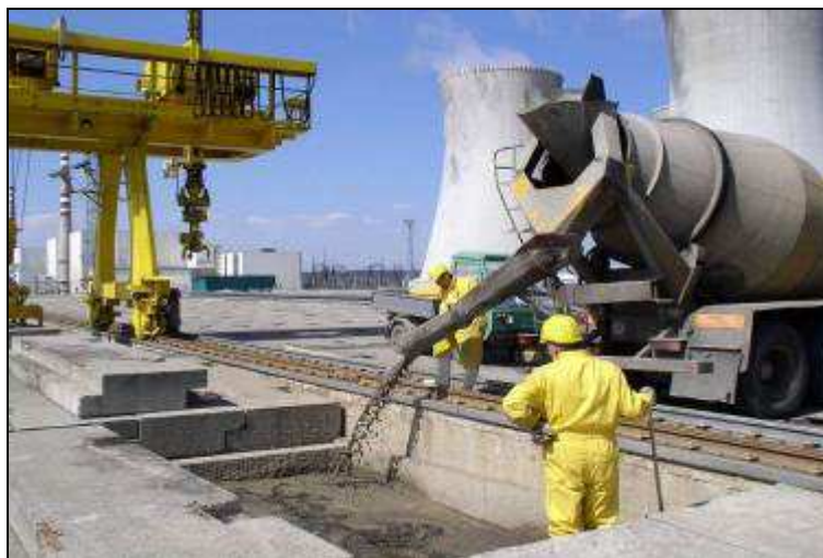
Fig. 8.3 Closing a full vault with concrete
