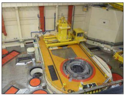
Fig. 4.1 SF pool and transfer cask shaft during reactor refuelling
