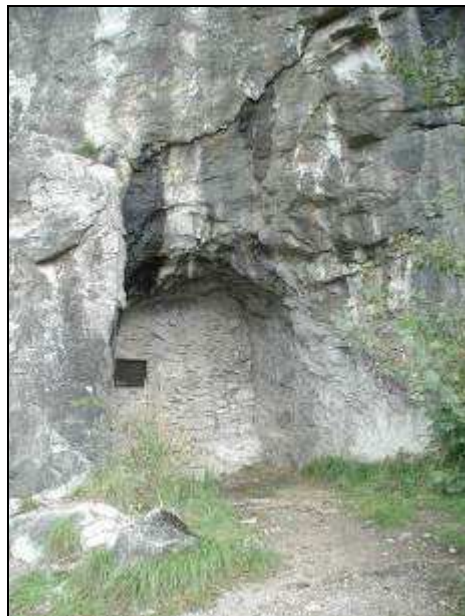
Fig. 8.5 Secured entrance into the RAW Disposal Facility Hostim
