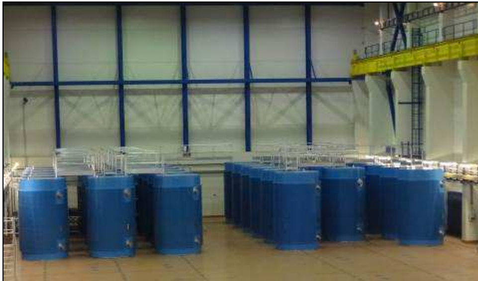
Fig. 4.2 Storage hall in SFSF Dukovany
