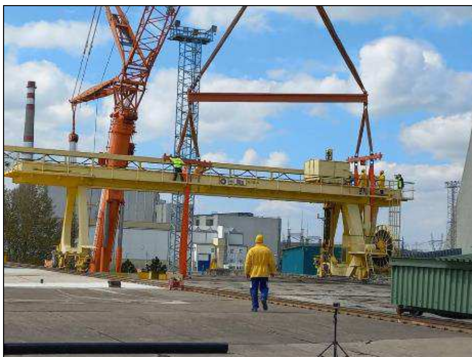
Fig. 8.3 Moving the gantry crane to the adjacent row
