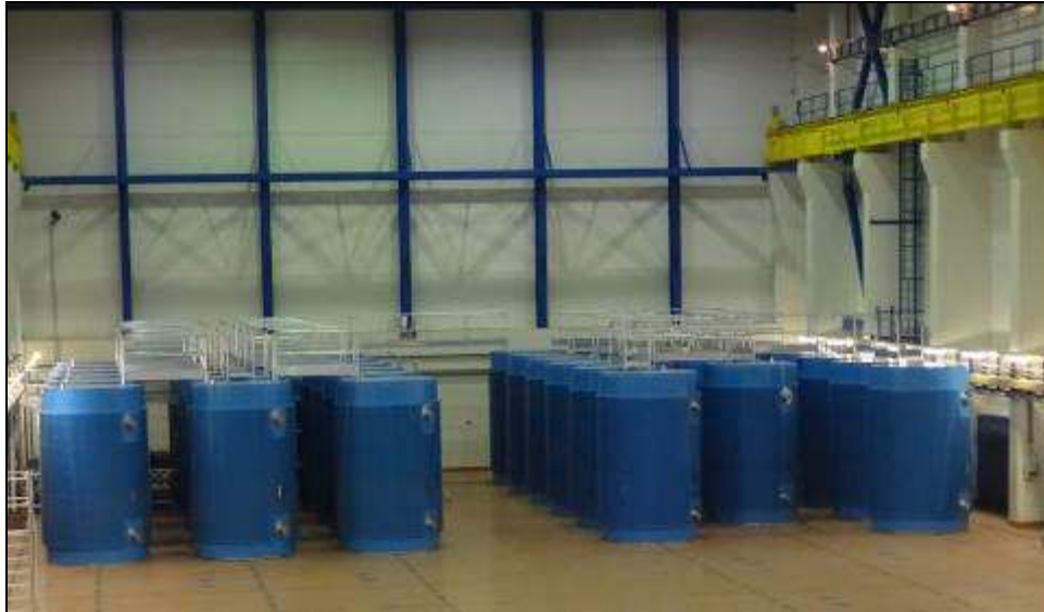
Fig. 4.2 Storage hall in SFSF Dukovany
