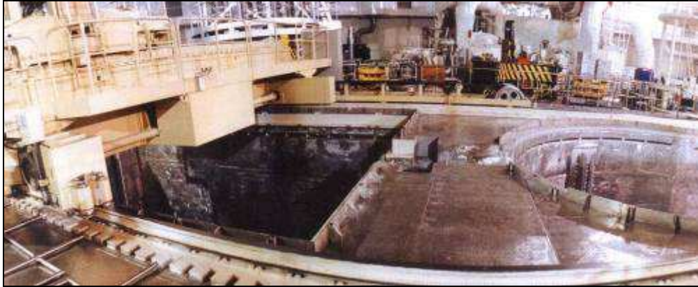
Fig. 4.3 Uncovered SF pool at NPP Temelín
